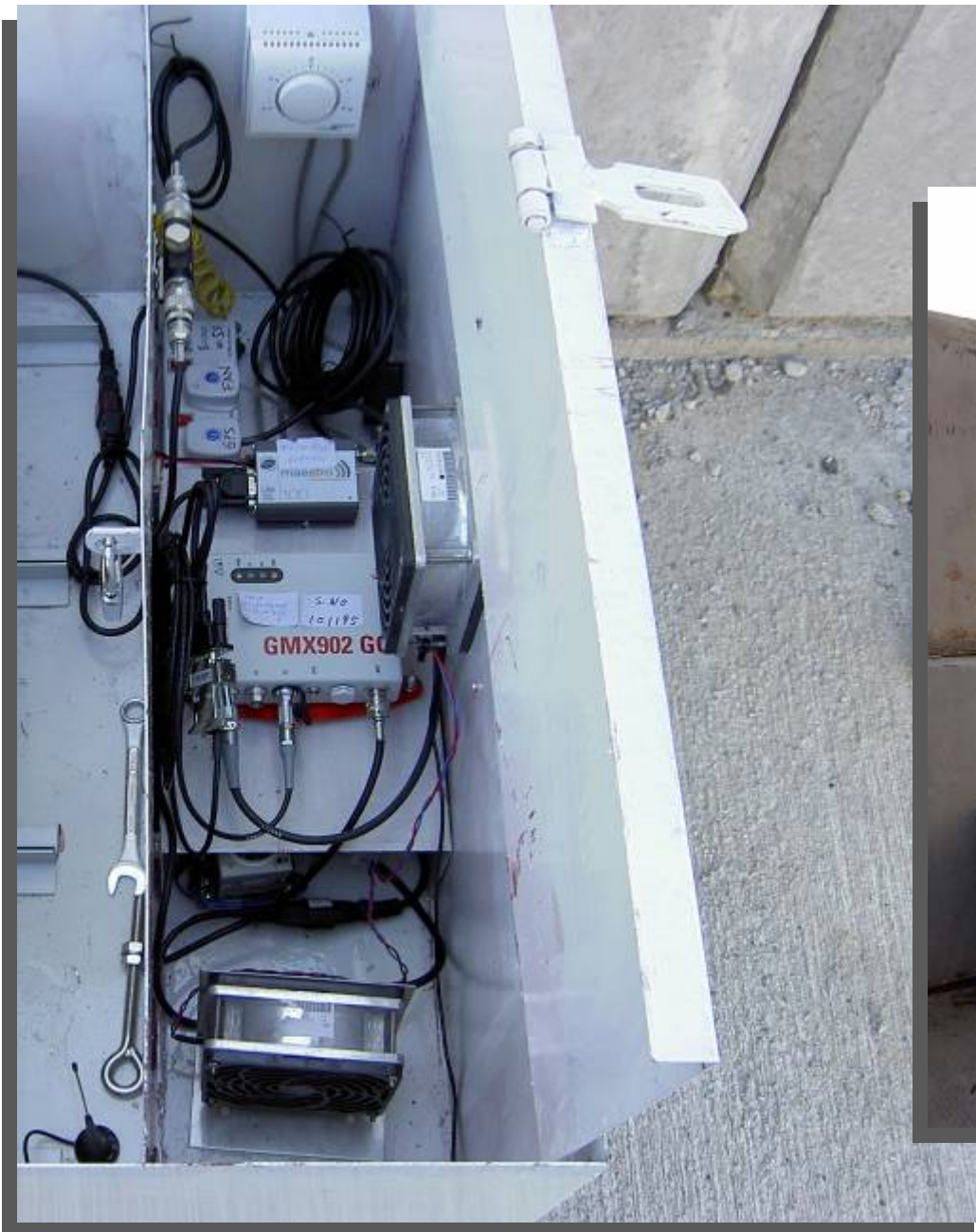
GNSS equipment, GPRS modem, power supply being installed inside a cabinet
