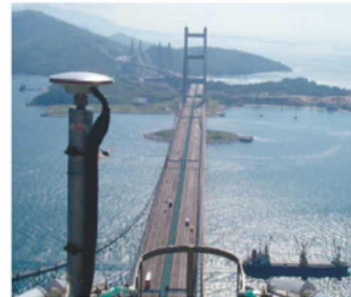
Receiver atop Tsing Ma Bridge tower, with Kap Shui Mun Bridge in the distance
