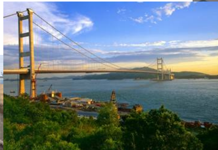
Bridge vibration & health monitoring
